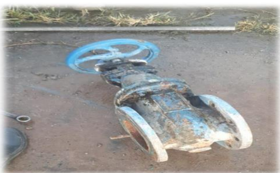
Removal of pump and valve
