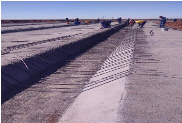
Construction of Drybeds
